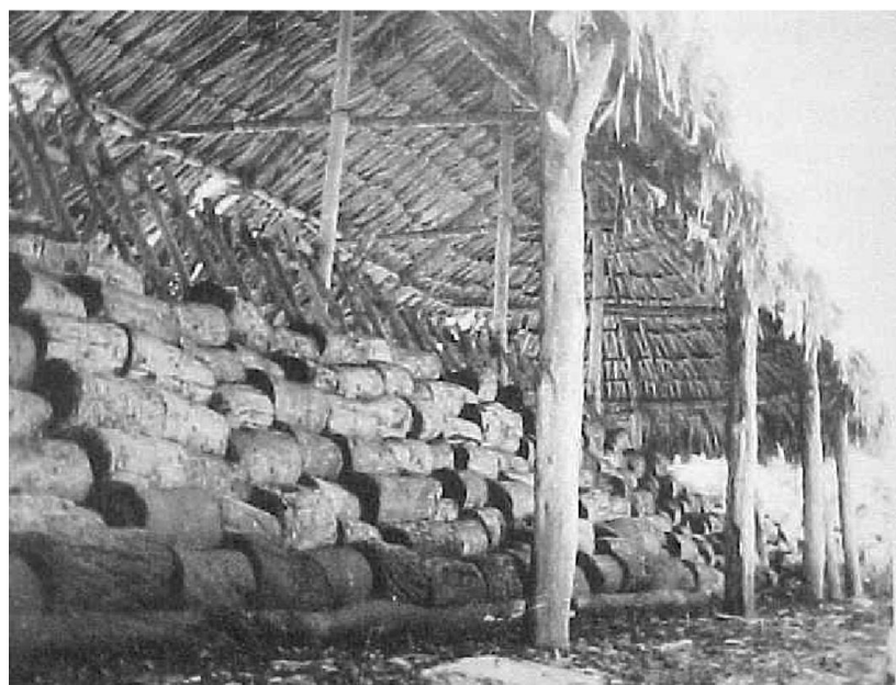
Figure 1: View of one of two sides of a traditional Maya meliponary from the beginning of the 20th century with several hundred hives (photo courtesy of Felipe Martínez López)
